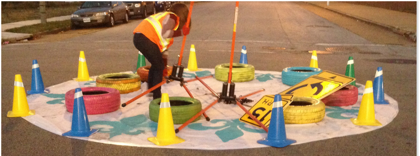
INSTALLING THE TEMPORARY MINI-ROUNDABOUT
