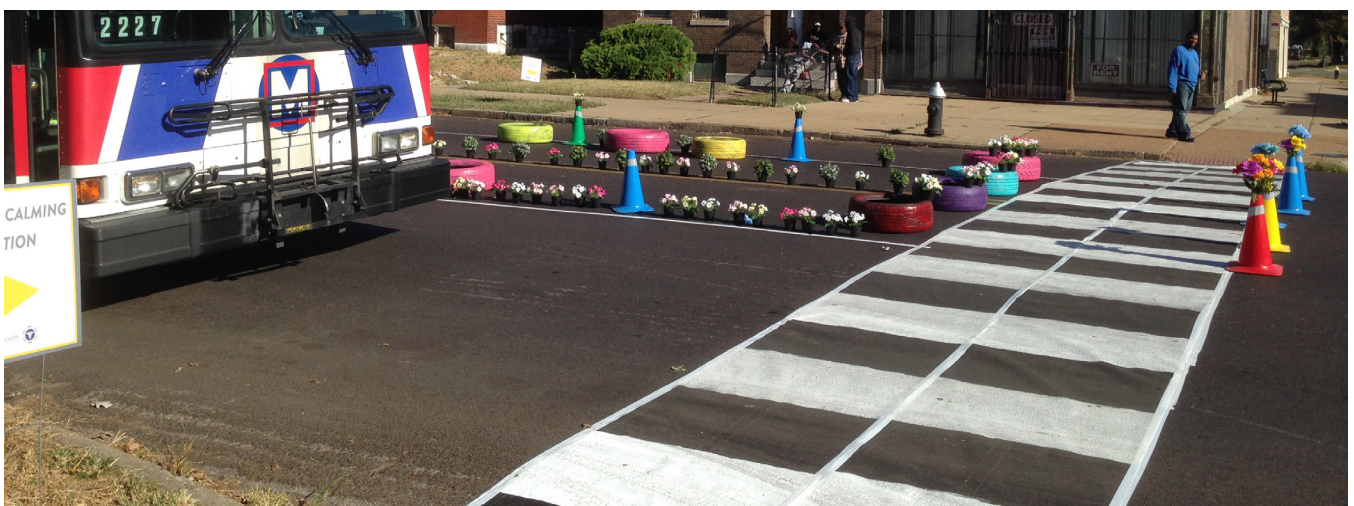
THE TEMPORARY CROSSWALK INSTALLED
