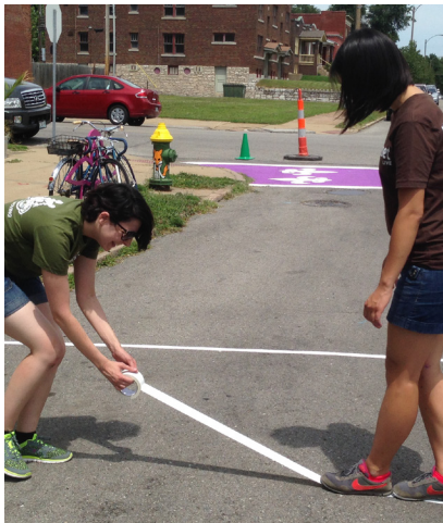
TRAILNET STAFF INSTALLING A TEMPORARY CROSSWALK
