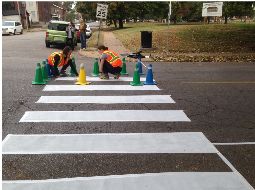
VOLUNTEERS INSTALLING TEMPORARY CROSSWALK
