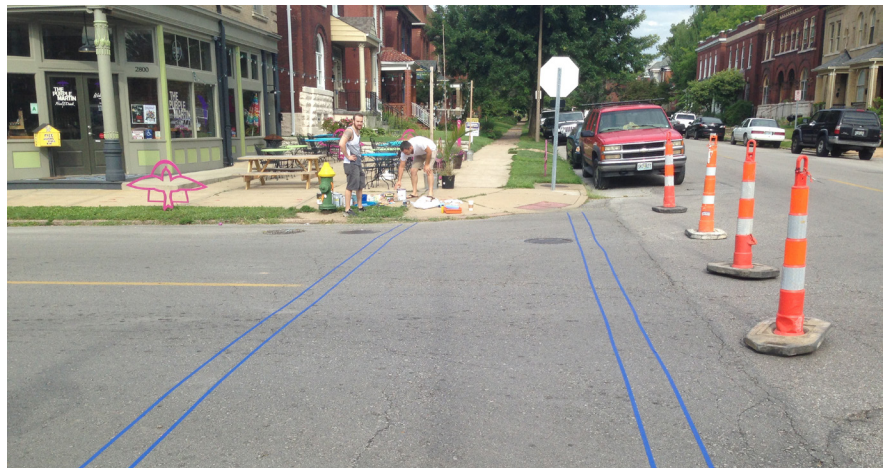
INSTALLING CROSSWALK ON DEMONSTRATION DAY
