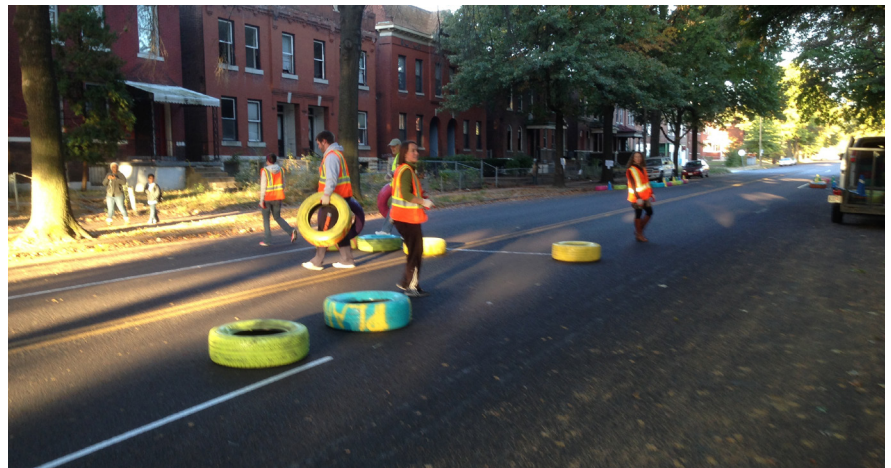
INSTALLING TIRES AND CONES ON DEMONSTRATION DAY
