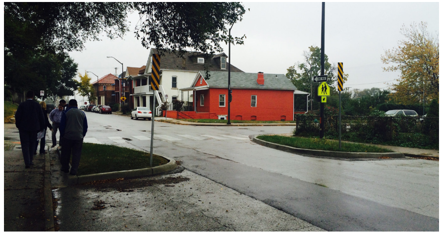
PERMANENT CURB EXTENSIONS CREATING NARROW LANES
