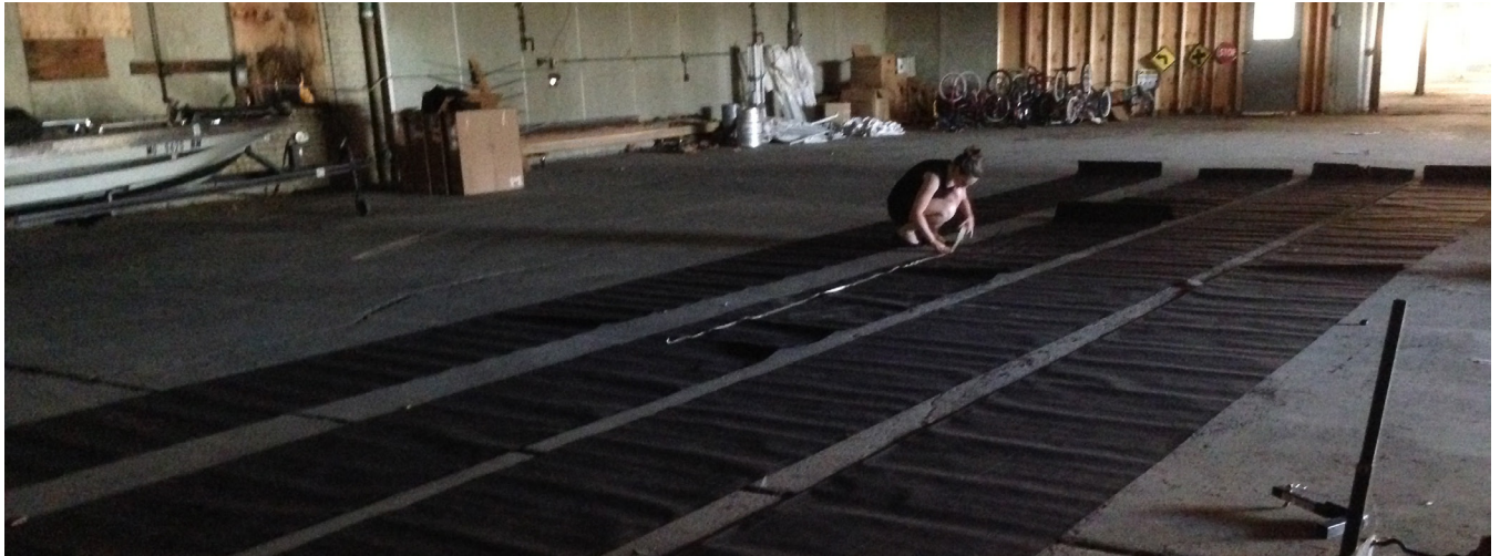
PREPARING TO PAINT THE TEMPORARY CROSSWALK
