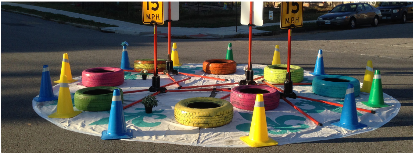
INSTALLING THE TEMPORARY MINI-ROUNDABOUT
