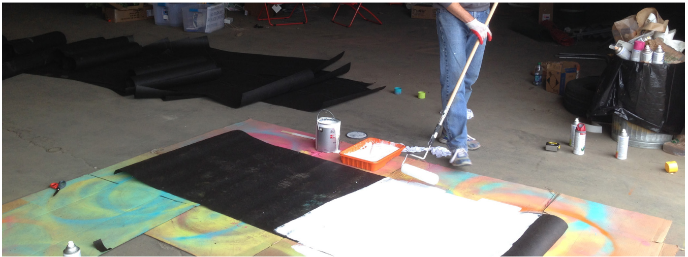
PAINTING THE TEMPORARY CROSSWALK
