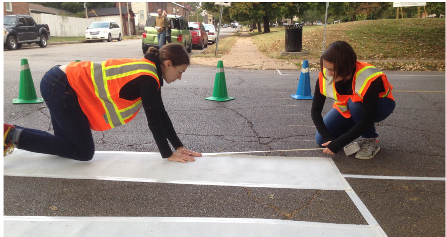
INSTALLING CROSSWALK ON DEMONSTRATION DAY
