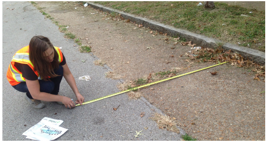
INSTALLING CHICANE ON DEMONSTRATION DAY
