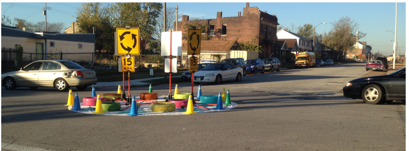
TEMPORARY MINI-ROUNDABOUT IN USE ON DEMONSTRATION DAY
