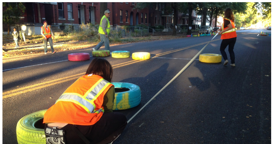
INSTALLING MEDIAN ON DEMONSTRATION DAY
